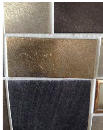
The severe scratching shown is typical of the damage caused by improper grout selection and grouting procedures.
