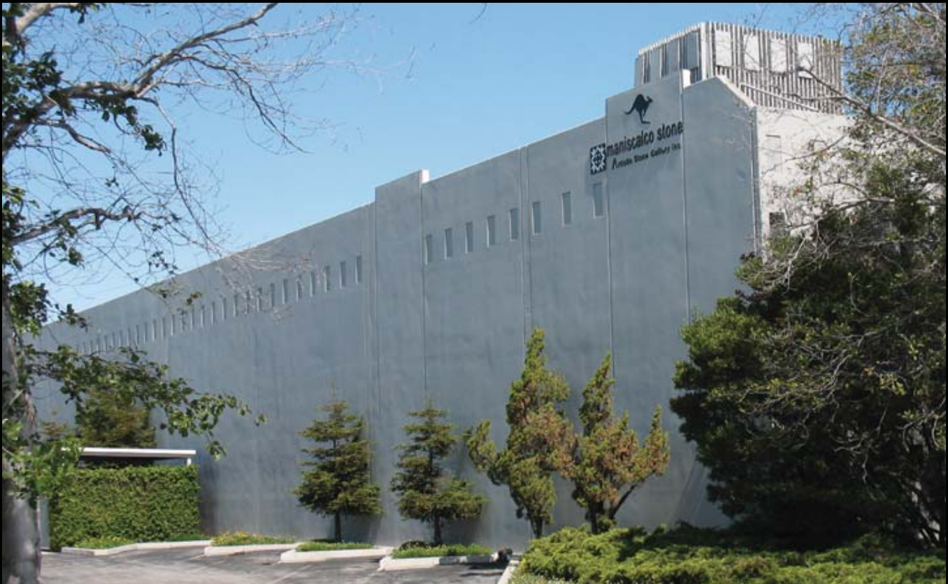
Maniscalco Head Office Menlo Park, California USA
